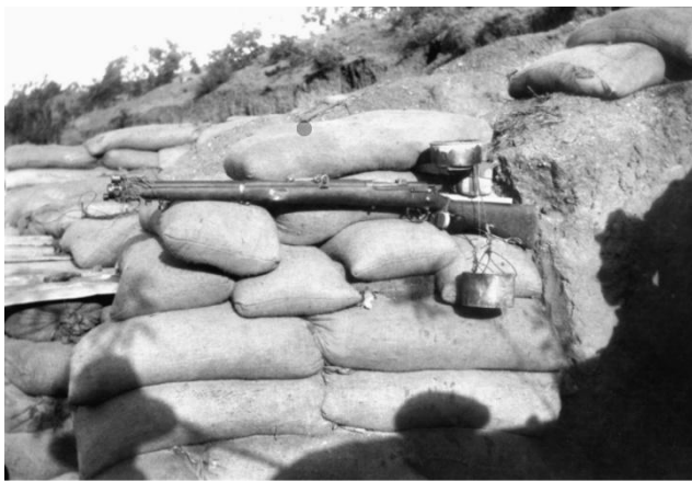
Figure 4. A drip rifle left behind to fire long after its owner had departed. Anzac ingenuity deployed in silence, 17 December 1915. Photograph by C.E.W. Bean, Australian War Memorial, accession G01291.
